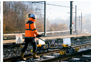
Rail Road Inspection
