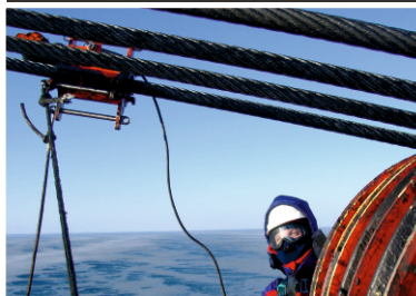
Wire Rope Inspection
