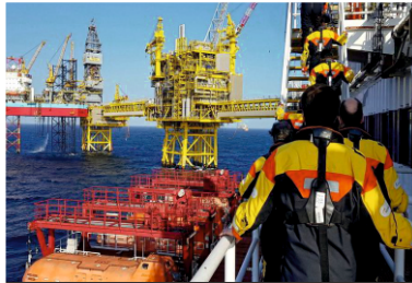
Offshore Platform Inspection
