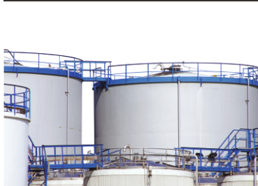
Storage Tank Inspection
