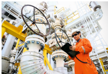
Pipeline Project Inspection
